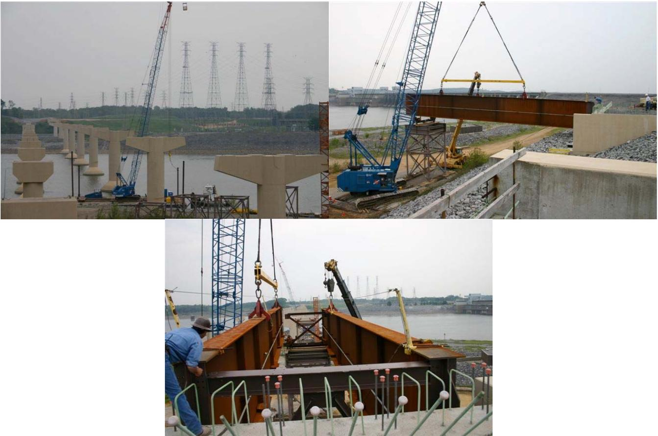
These are girders for the new highway bridge across the TN River below KY Dam – being erected on piers constructed under a previous contract. US Hwy 62 is being relocated off the dam to make room for the new lock. Later this summer, girders will be installed for the new RR bridge that is just 100 feet downstream from this Hwy bridge. This work is part of the \$96M Superstructure Contract that complete the RR and Hwy relocations.
